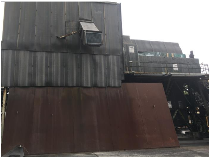
Plate 4.7 Noise mitigation cladding on CHPP
